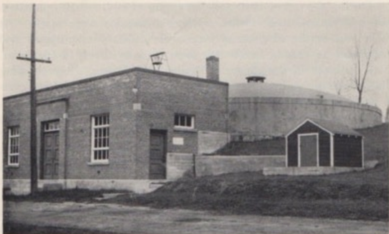
View of pump-house, 200,000-gallon water storage tank, and housing for new deep well.
